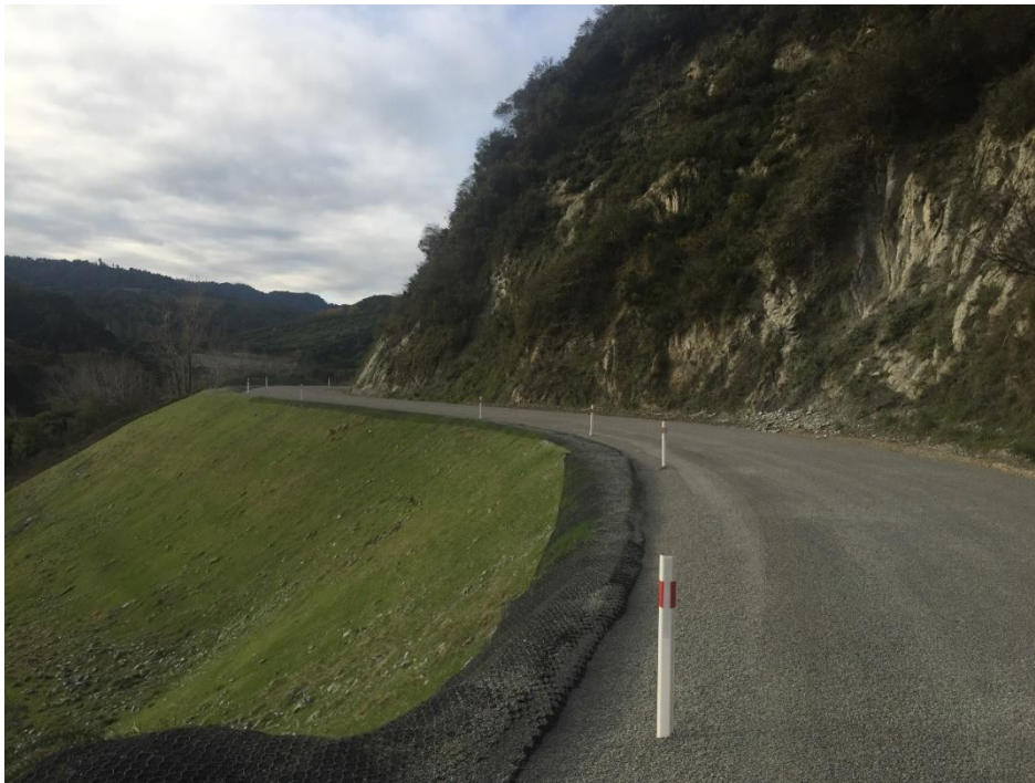
Photo: Completed sealed road surface, above Kauwaeroa Dropout site
