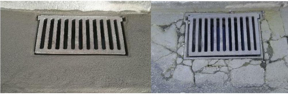
Before and after - Repairs to the bus stop outside St Josephs School, Mcphee St, Dannevirke
